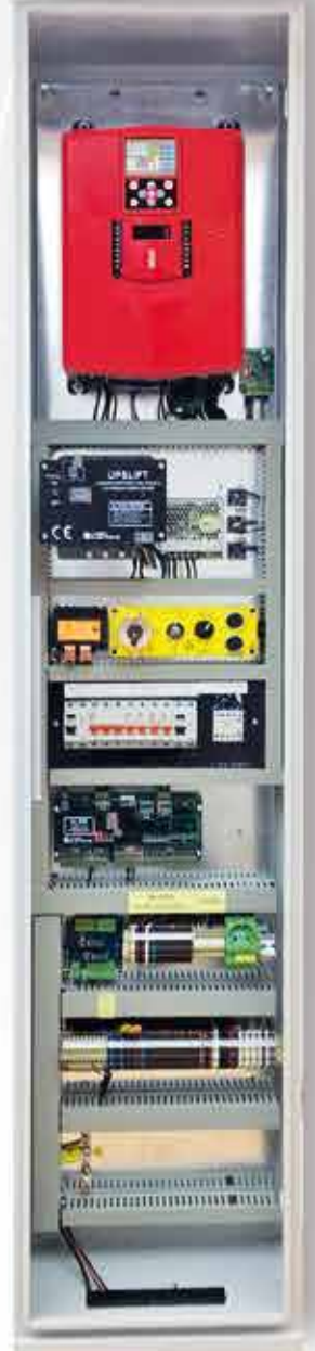
MRL Control Panel
